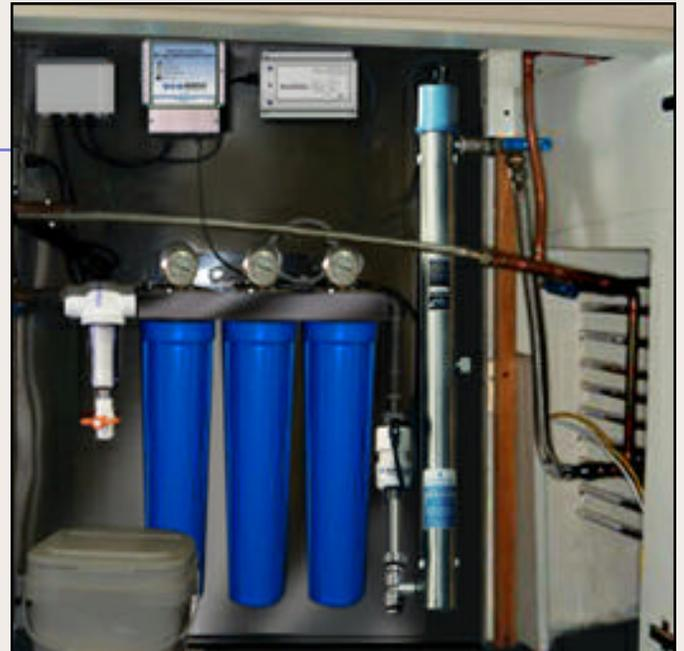
Multi-Process factory integrated All-In-One modular unit, filtration, deposit control, ultra-violet disinfection & purification installed at a dental facility (end-to-end treatment & conditioning).
