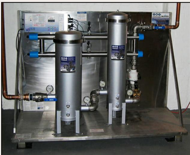
Skid-mounted Multi-Process factory integrated All-In-One modular unit, filtration, deposit control, ultra-violet disinfection & purification installed at a multi-dwelling residential facility.
