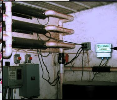
Deposit controller and on-site solenoid coil application
